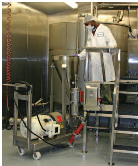
Powdered glucosamine and chondroitin are predispersed in a liquid stream of filtered water. This in-line SLIM mixer replaced a batch mixer and serves two 1500-gallon vessels. Photos courtesy of Botanical Laboratories.
